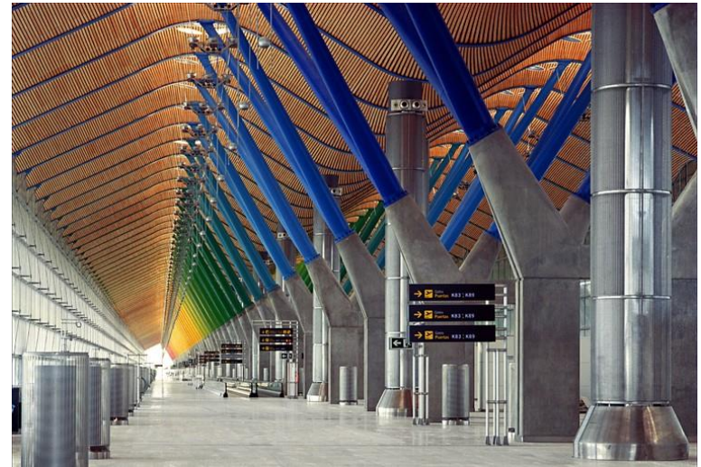
Madrid-Barajas Airport Terminal 4 / Estudio Lamela & Rogers Stirk Harbour + Partners
